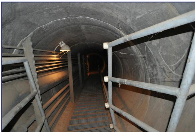
*A tunnel leads deep into the original Exchequer Dam, now submerged under Lake McClure. Part of its infrastructure is still used for power production at New Exchequer Hydroelectric Project.*
