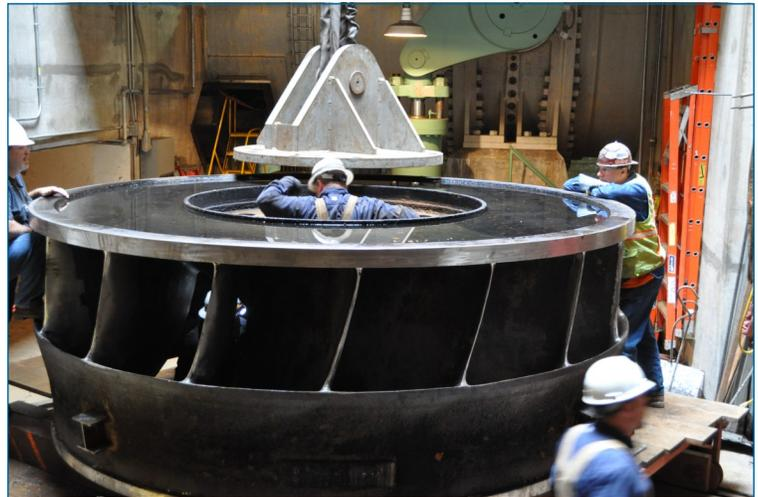
Workers inside the bottom of New Exchequer dam prepare to attach a "runner" to a crane so it can be removed from the powerhouse. The runner is a propeller-like component that spins as water rushes past it and turns a generator to produce emission-free electricity.
