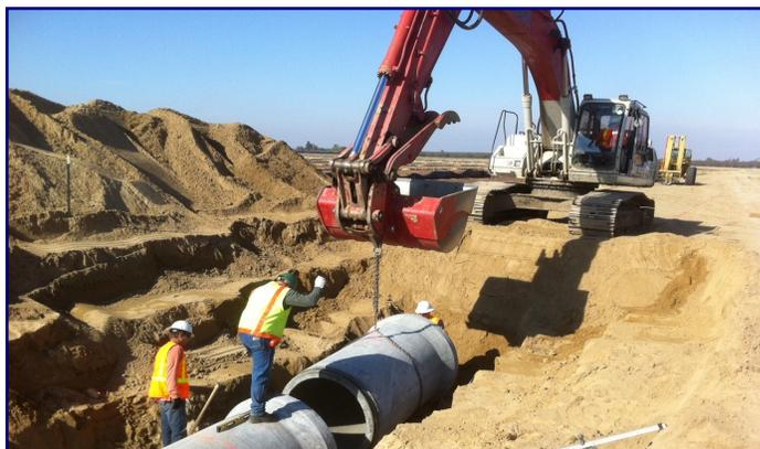
Workers install pipeline as part of the Garibaldi Lateral Water Conservation Project. By connecting two canal laterals west of Livingston, the project will allow approximately 5,600 acre feet of irrigation water to remain in MID's canals each year that would otherwise spill to the Merced River.
