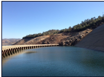
The original Exchequer Dam, above, was constructed in the 1920s. It has mostly remained submerged after the larger New Exchequer Dam was constructed just downstream in the 1960s. The original dam is visible, at left, in the shadow of the larger New Exchequer Dam after two dry years.
